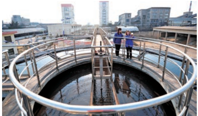
Mine water efficiency sedimentation basin
